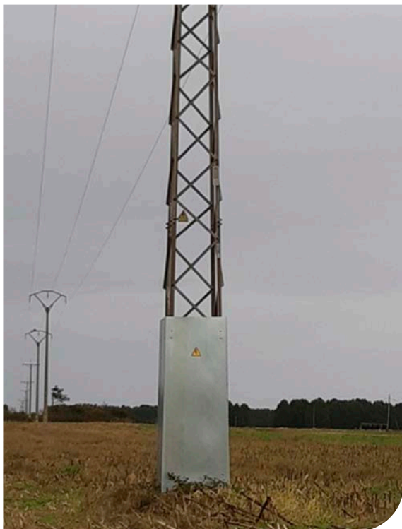
Foto antes obra. Photograph taken before the start of the works.
