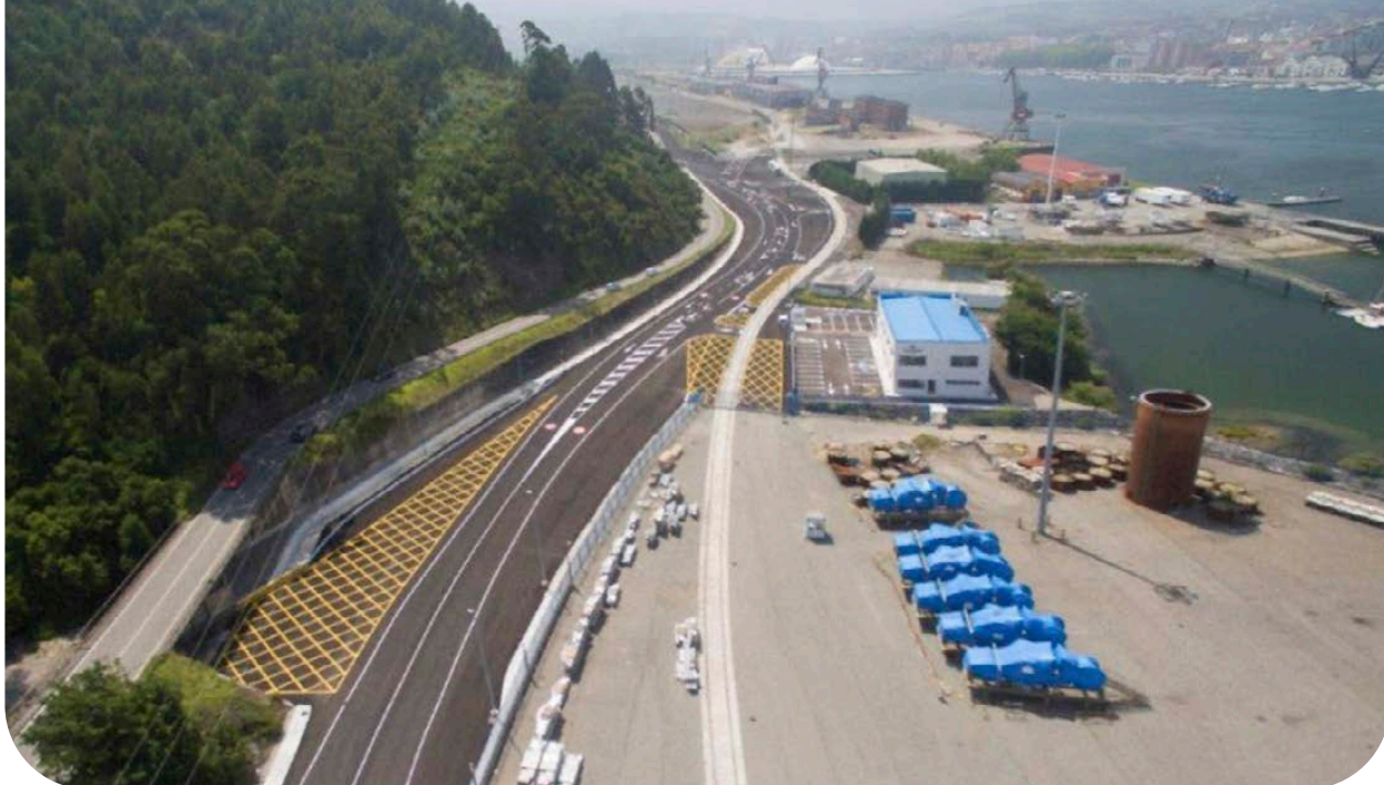
Vista aérea del estado final de las obras. Julio de 2021. Aerial view of the works upon their completion. July 2021.
